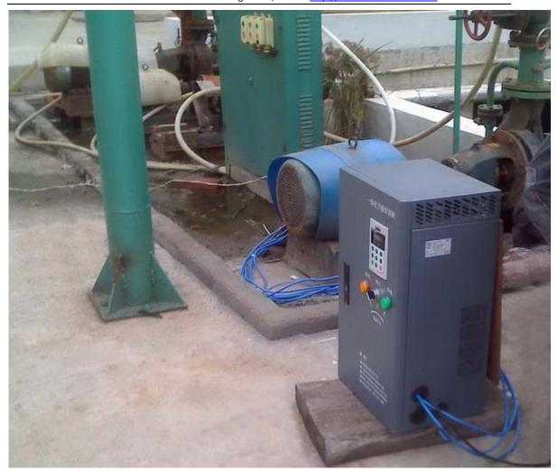
PID feedback closed loop control & vector control variable speed drives (AC drives, frequency inverters) for constant pressure water supply
